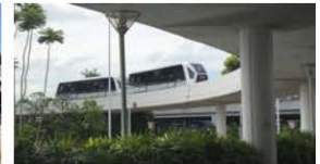
Changi Airport Skytrain APM Guideway, Singapore
