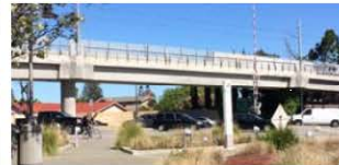
VTA Hamilton Station Viaduct Guideway
