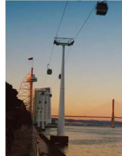
Telecabin Lisboa Cable Guideway Tower, Lisbon, Portugal
