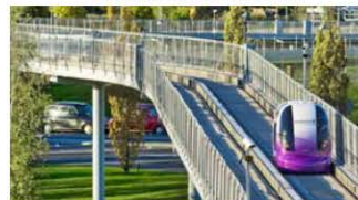
Heathrow Airport PRT Guideway, London, UK
