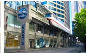
Seattle Monorail Guideway
