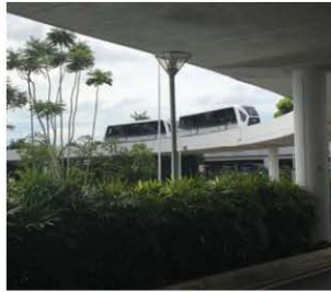
Changi Airport Skytrain APM Guideway - Singapore
