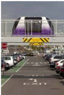
Heathrow Airport PRT Guideway - London, UK
