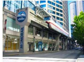
Seattle Monorail Guideway
