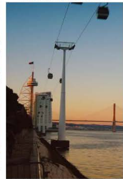
Telecabine Lisboa Cable Guideway Tower - Lisbon, Portugal
