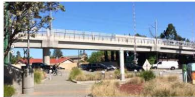
VTA Viaduct Guideway
