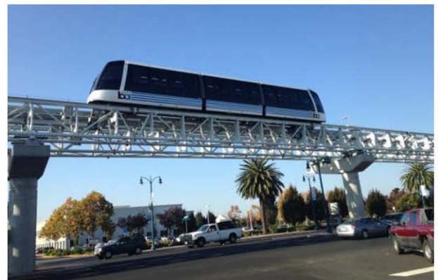
Doppelmayr Cable Car: Cable Liner (Oakland, CA)
