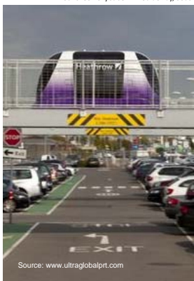
Heathrow Airport PRT Guideway, London, UK
