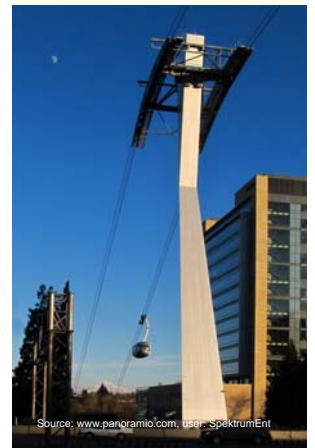
Portland Aerial Tram Cable Guideway Tower
