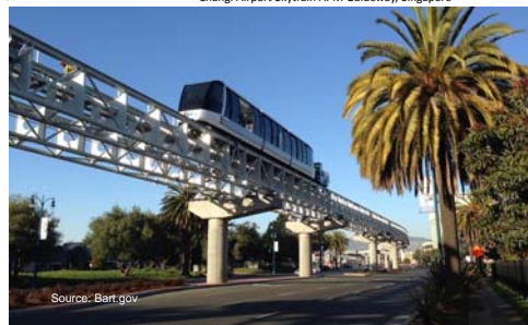
Oakland Airport Connector APM Guideway
