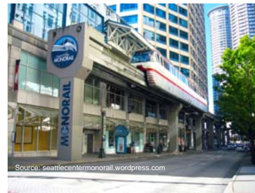
Seattle Monorail Guideway
