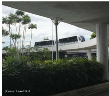
Changi Airport Skytrain APM Guideway, Singapore
