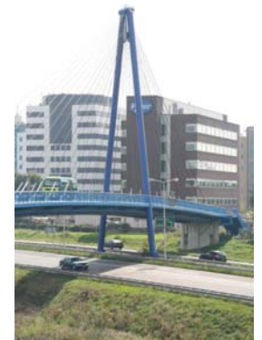
Rivium GRT Guideway, Netherlands
