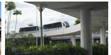
Changi Airport Skytrain APM Guideway, Singapore
