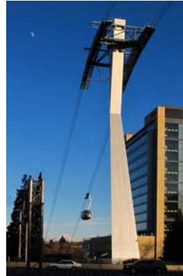
Portland Aerial Tram Cable Guideway Tower
