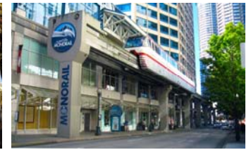
Seattle Monorail Guideway
