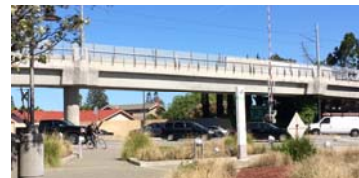
VTA Hamilton Station Viaduct Guideway
