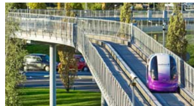
Heathrow Airport PRT Guideway, London, UK
