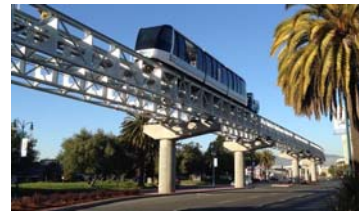
Oakland Airport Connector APM Guideway
