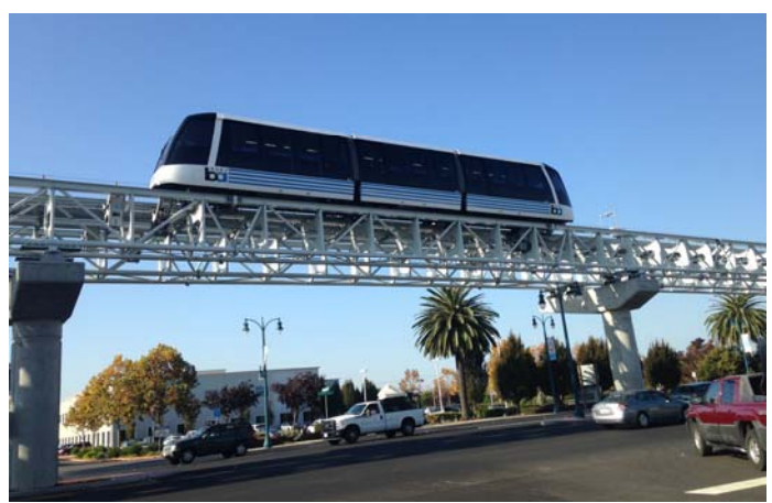
Doppelmayr Cable Car: Cable Liner (Oakland, CA)
